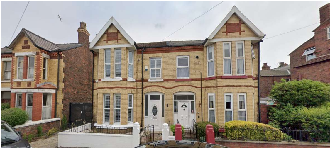
No's 2 & 4 Somerville Road opposite the site (above)
