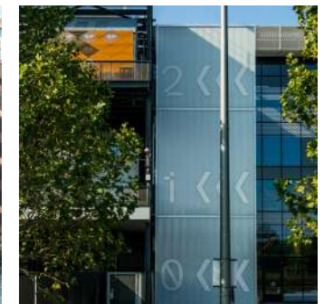
Clear signage for a multi-storey car park
