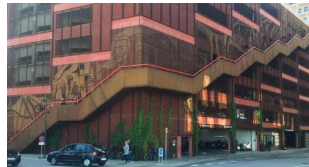
Example of a bespoke car park with natural green walls and place specific imagery on the exterior to make attractive
