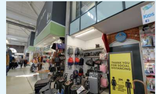
Heritage assets from the Market Hall are hidden behind plaster and stalls
